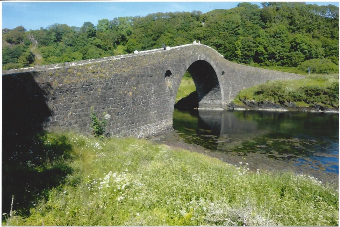
Clachan Bridge (Bridge over the Atlantic)
